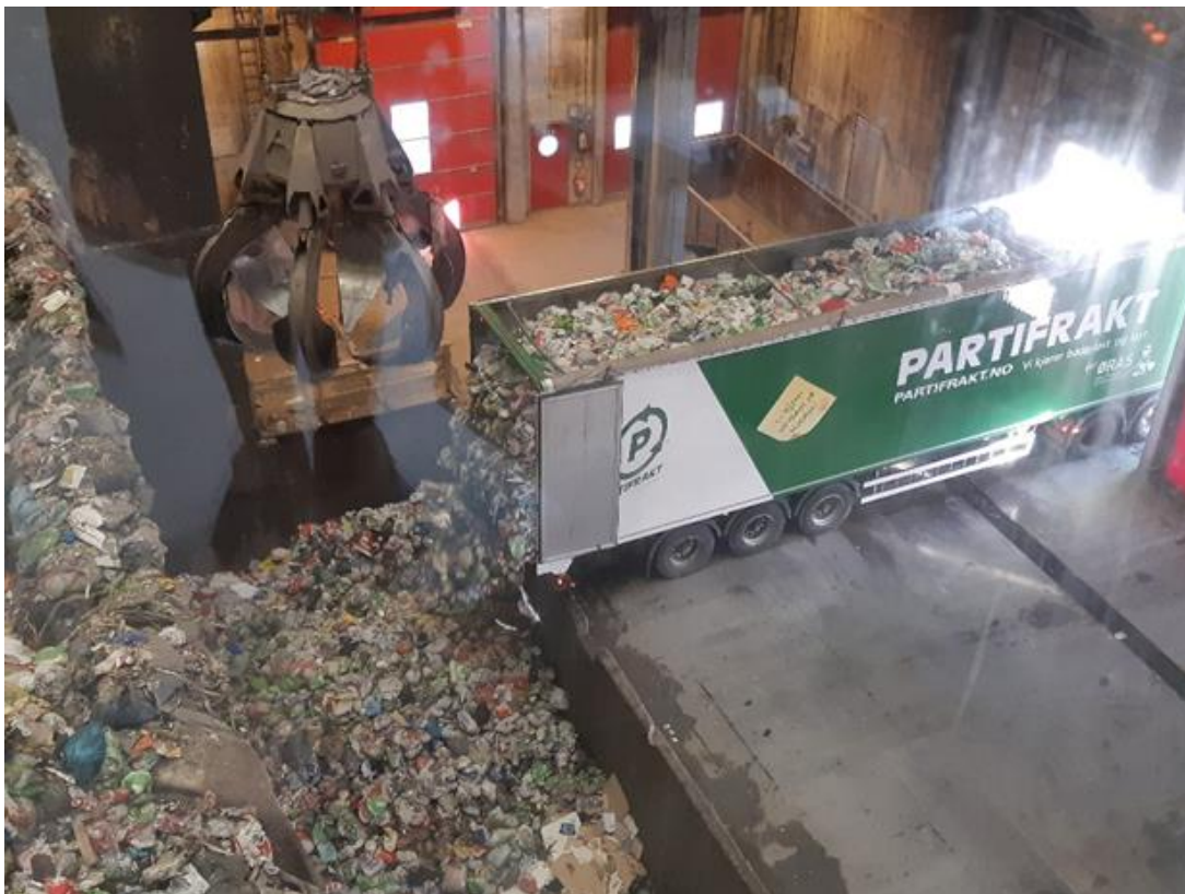
Figure 1. Unloading waste fuel from Norway into the fuel bunker.
