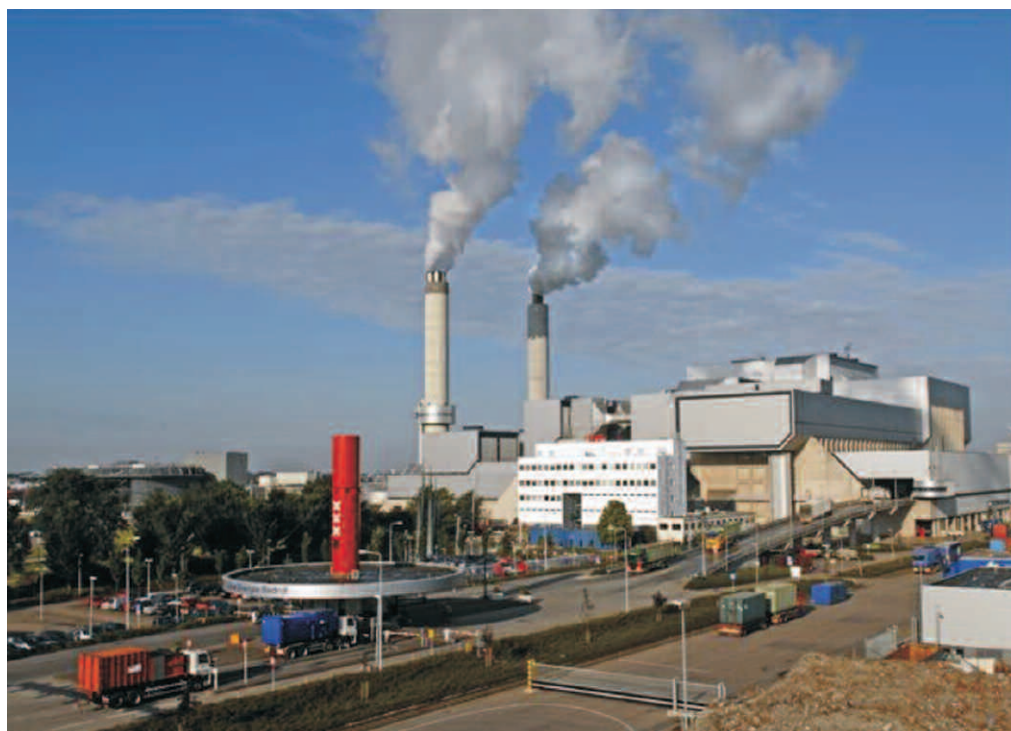
Waste Fired Power Plant® Amsterdam, photo courtesy of AEB.
