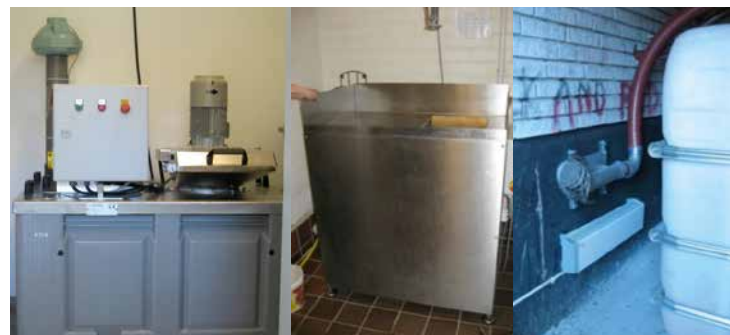
Figure 15: A grinder and a tank connected device (left). A simpler solution, with a grinder in the kitchen connected to the waste tank placed in a garbage room (right). (Source: Stockholm stad)
