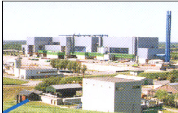
Figure 11. VAM waste incineration plant, Holland.
