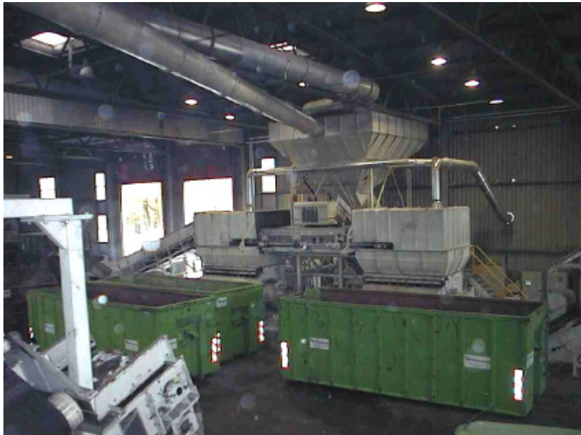
Figure 17. Secondary crushing of paper and plastic fraction.
