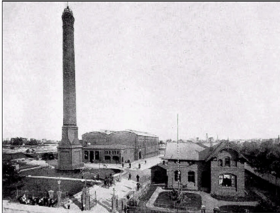
Fig. 8 First continental waste incinerator Hamburg Bullerdeich (1896)
