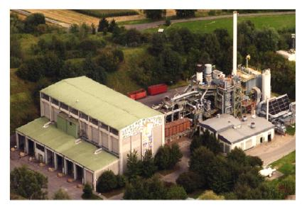
Capacity: 2 x 3 Mg/h Configuration: 1 X 2.2 MW CHP Process: pre-shredding, pyrolysis at 470 °C – 500 °C, pyrolysis-gas combustion at 1,250° C
