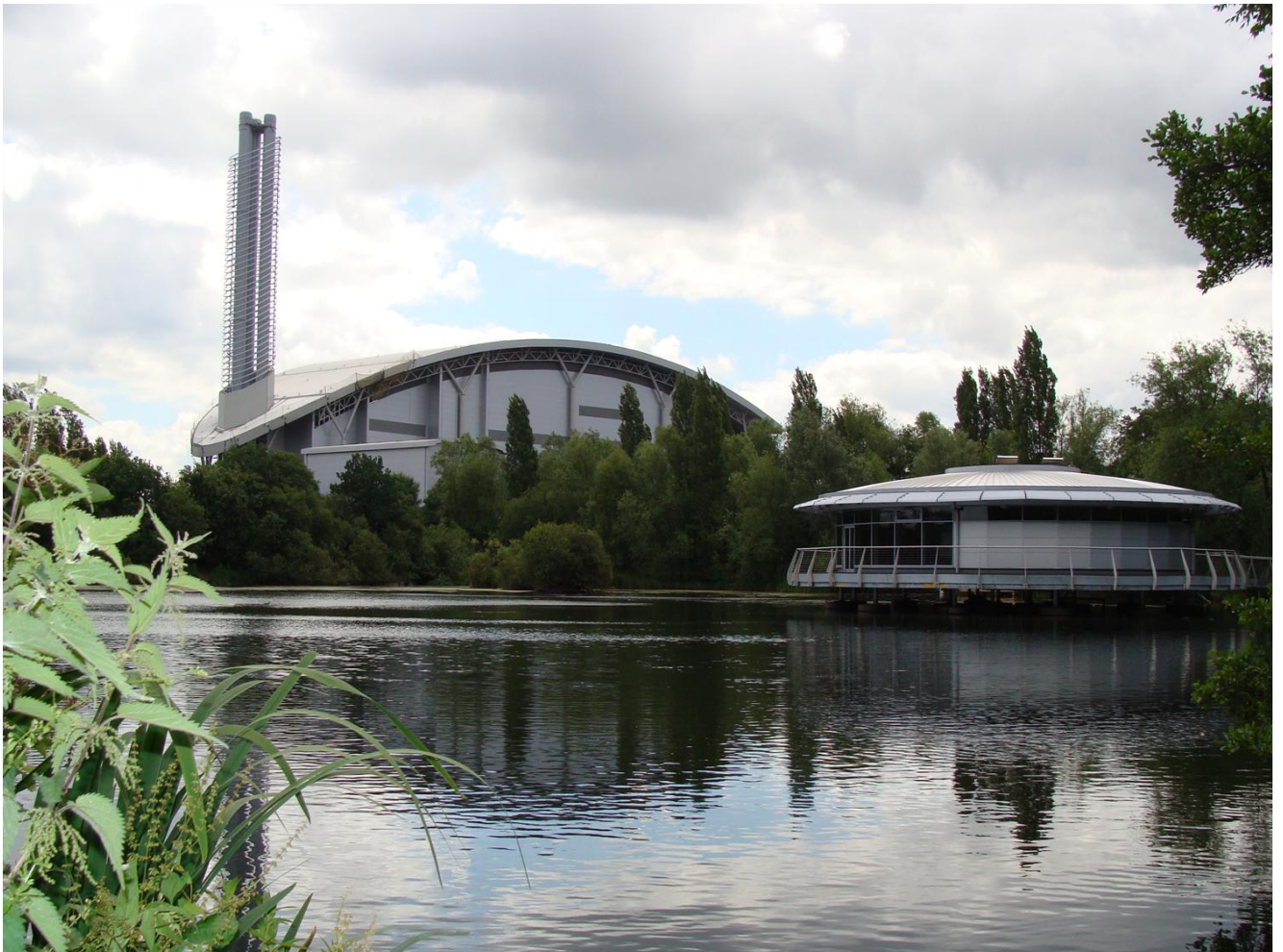
Lakeside Energy from Waste Plant, UK
