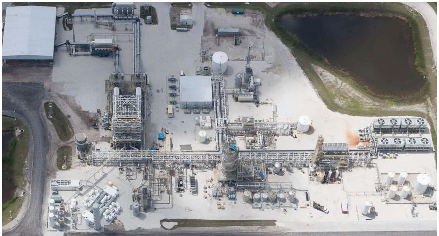
Figure 10 Ineos Bio's Vero Beach plant in construction, August 2012
