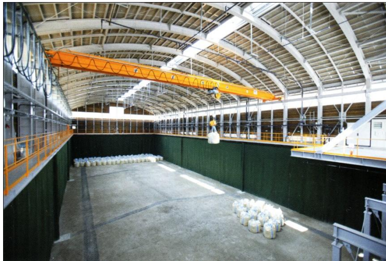
Figure A2.27: Pit for storage of APC residues
