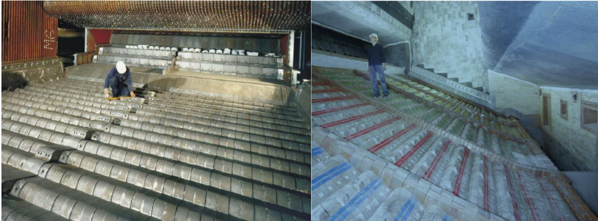
Figure 4.15: Combustion chamber with two lines of a horizontal grate (left) and five lines of a reverse-acting (right; adopted from [Martin 2009])
