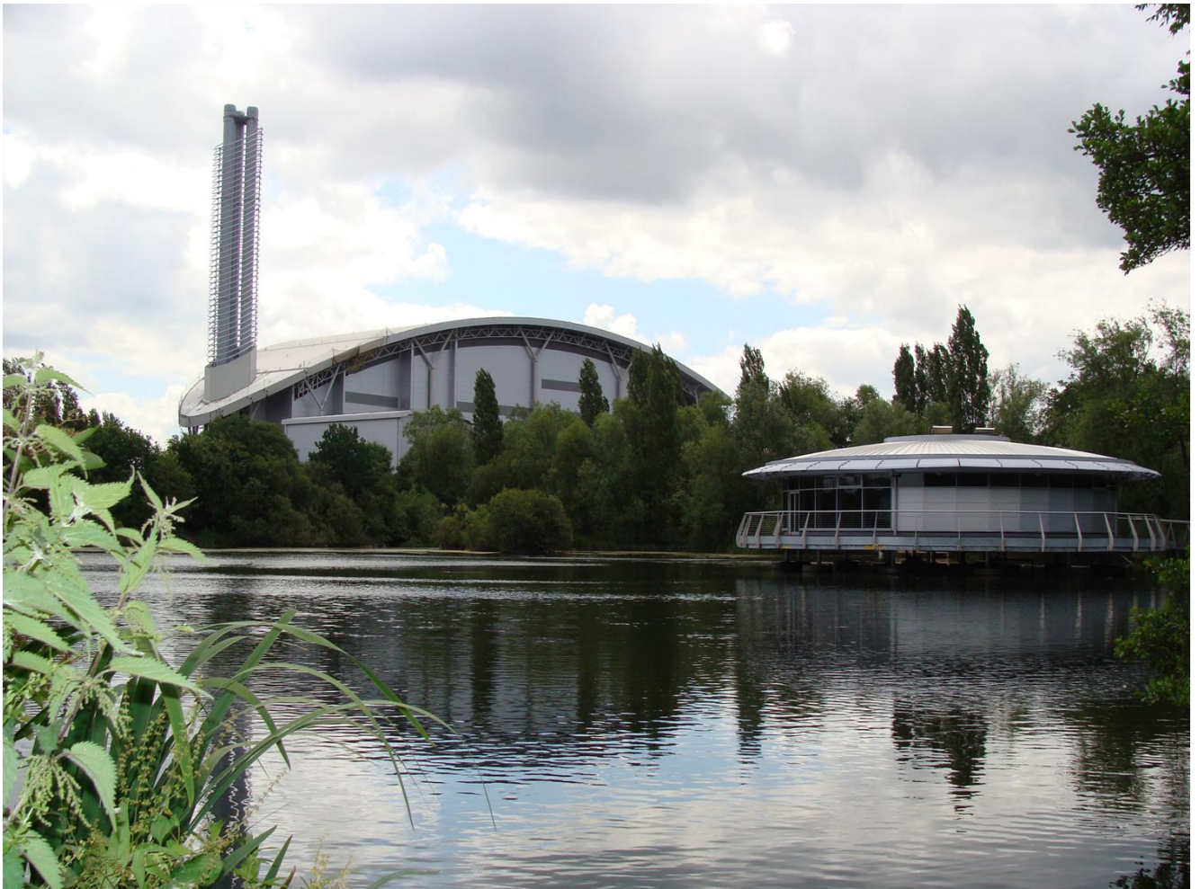
Lakeside Energy from Waste Plant, UK
