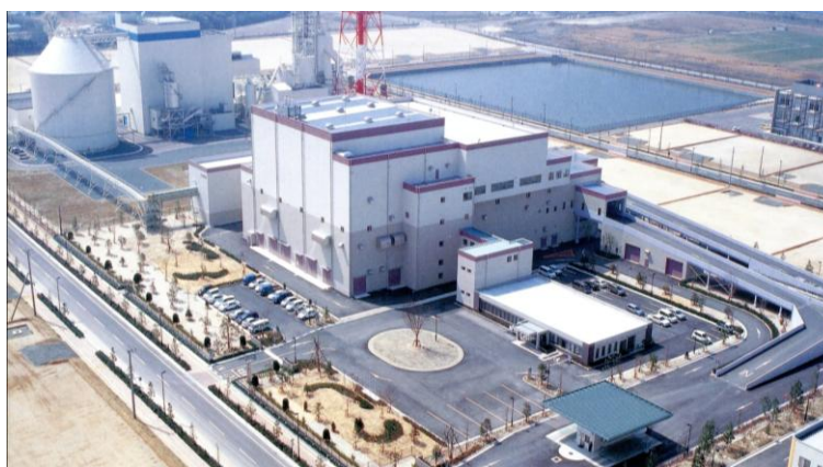
Figure A2.7: Aerial view of the Omuta-Arao RDF Center
