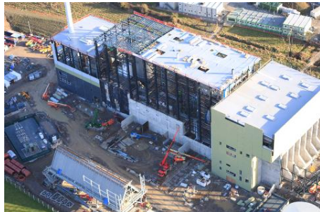
Commissioning Feb - Jun 2011
