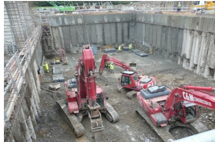
Foundations & Bunker Sep - Nov 2009
