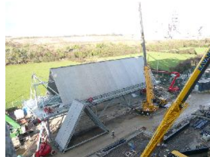
Turbine & air condensers Dec 2010
