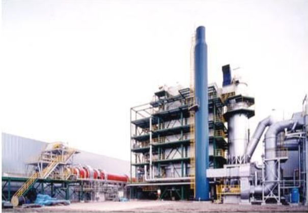
Takuma pyrolysis plant
